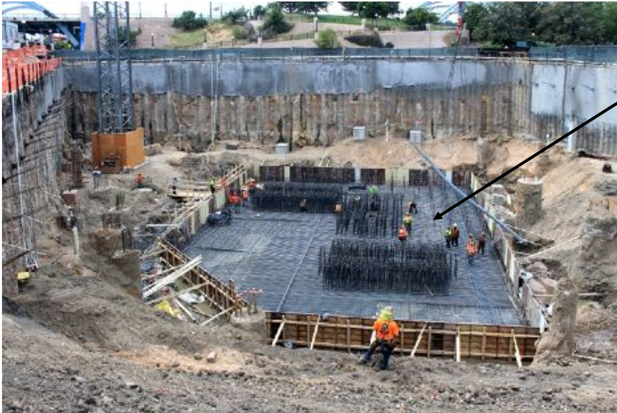
Tying Steel for the Shear Wall Mat
