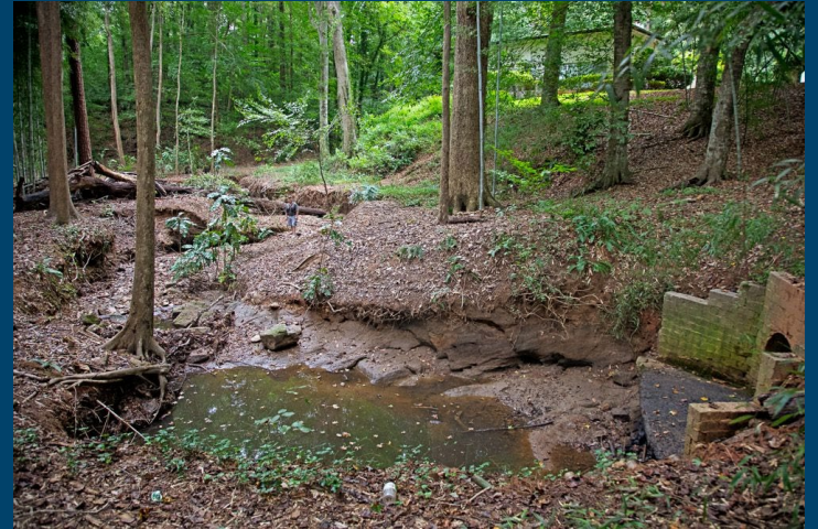
Minor-Moderate Erosion Stream Stabilization
